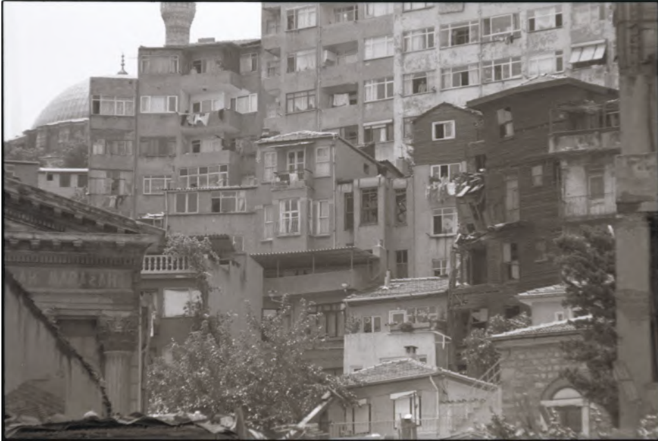
Figure 2: A View From Balat Streets, SALT Research, Eleonora Arhelaou Collection, 1989. Photographer: Eleonora Arhelaou. Title: Buildings number 20 and 22 on Usturumca Street
